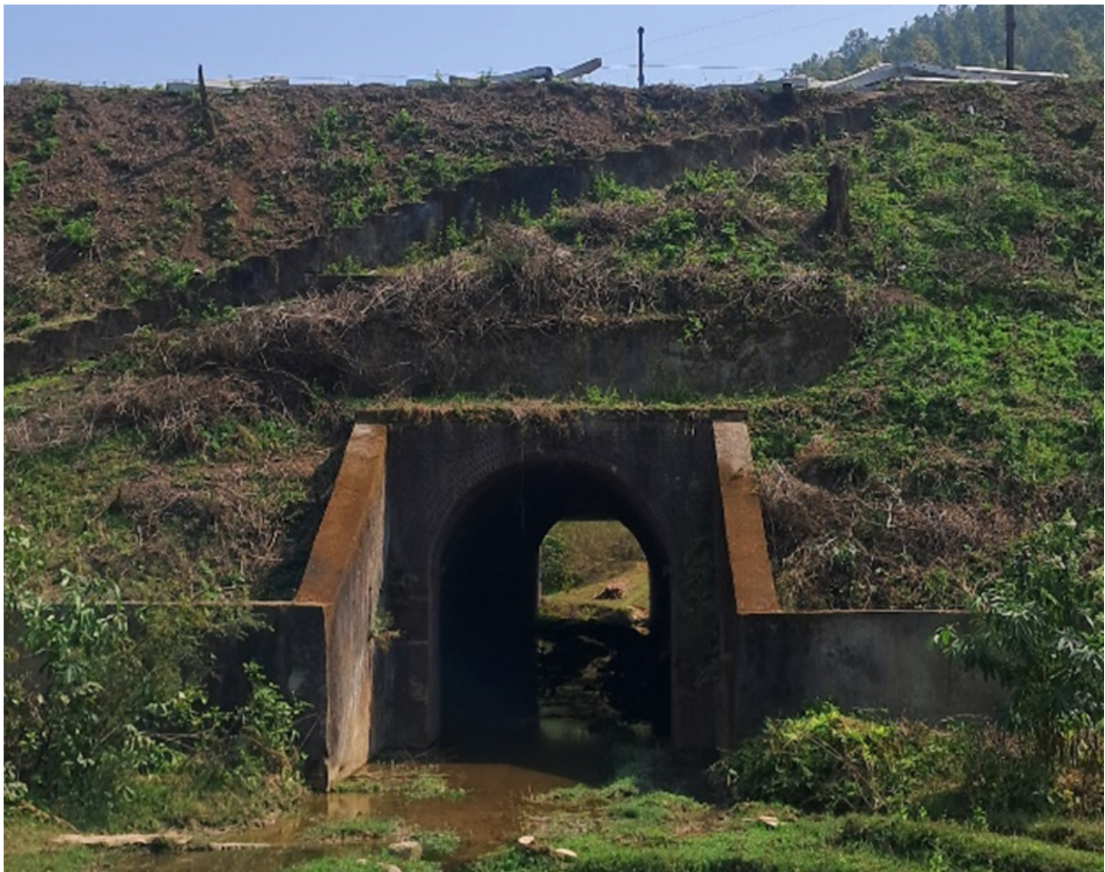
Figure 6: Existing culverts need structural modifications for elephant underpass
