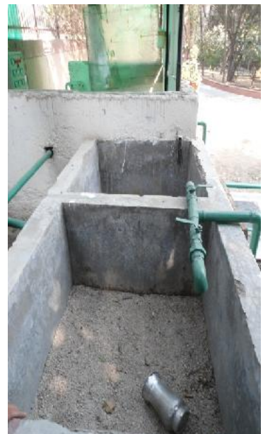
STP/ETP installed and the sludge drying bed without any sludge
