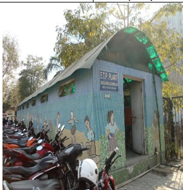
ETP Installed by the Hospital-Not operation
