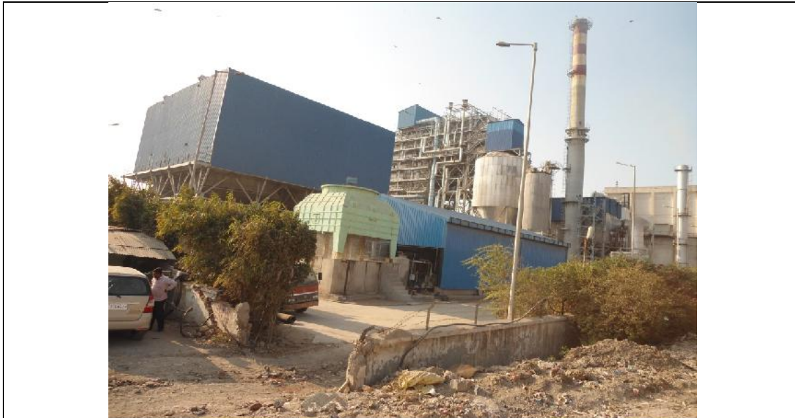
Waste to Energy Plant at Ghazipur
