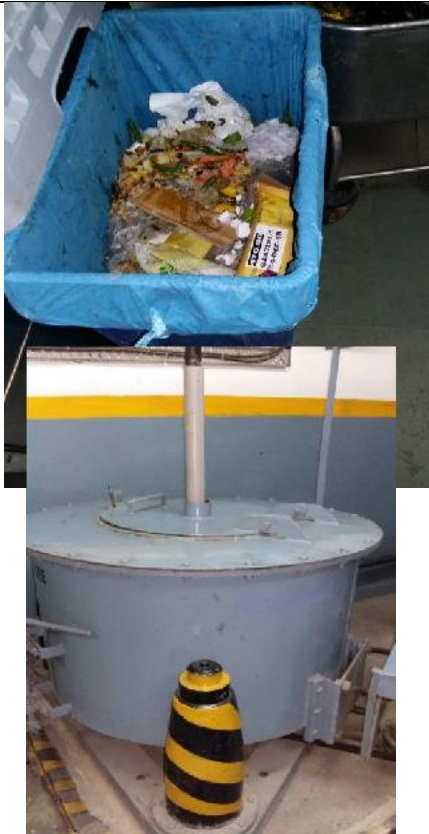
Mixed waste Storage Bin, On-site compost plant and the centrifuge as a part of STP
