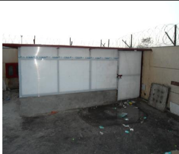
Temporary MSW Storage shed
