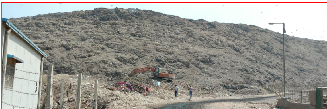
Fig.1 Typical view of Ghazipur MSW dumping yard
