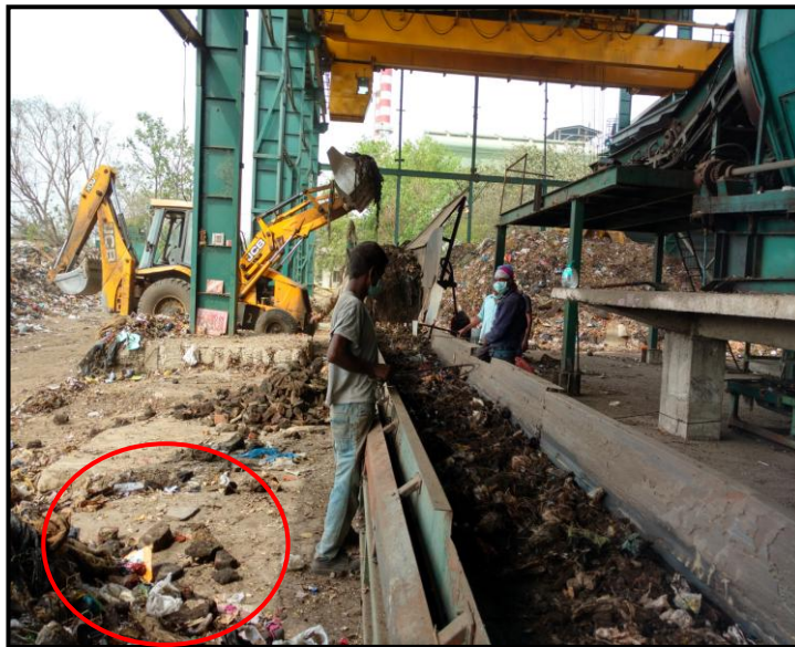
Fig.5:- Removal of Brick bats, C&D waste from the conveyor
