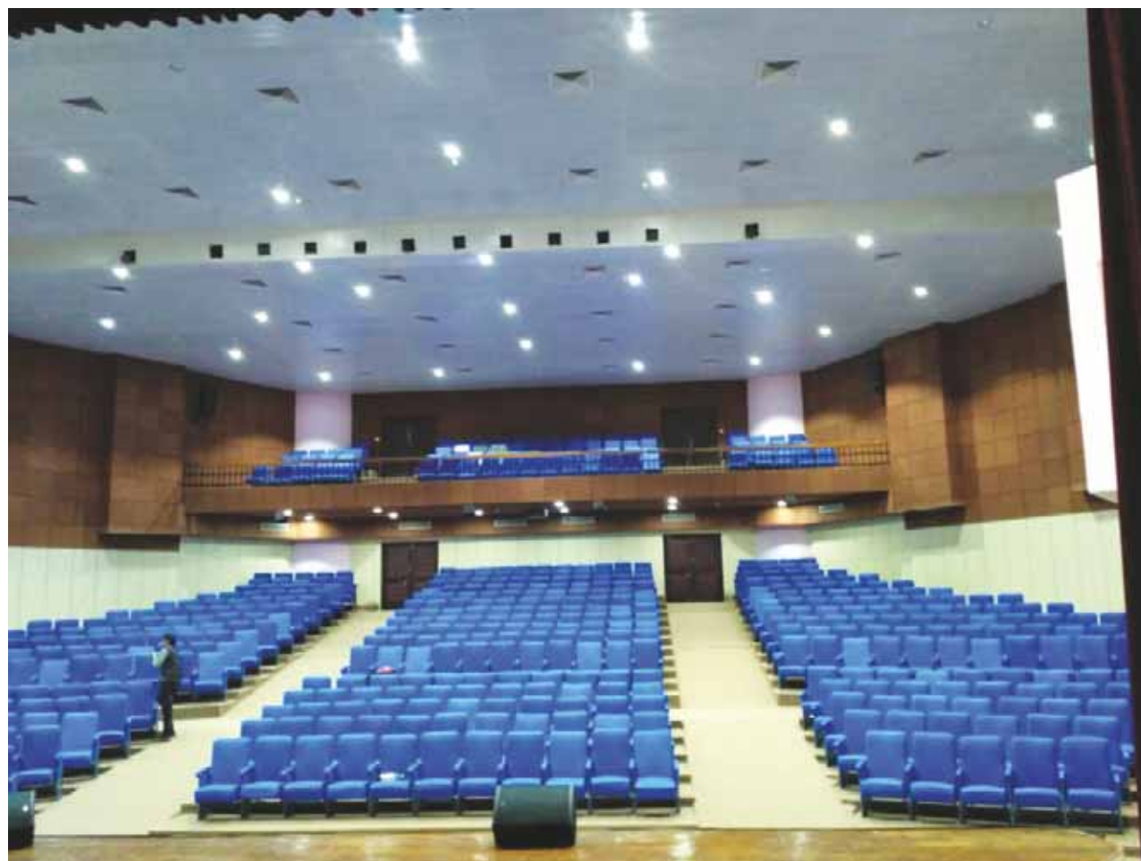
Fig. 79 Renovation of Hari Singh Auditorium for Indira Gandhi National Forest Academy (IGNFA), Dehradun
