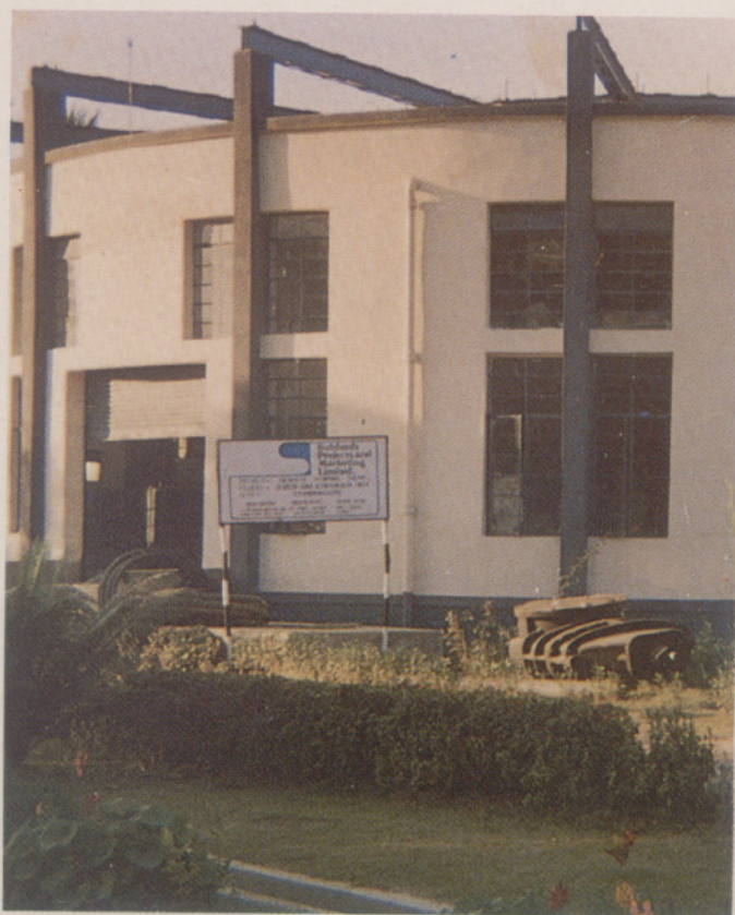
Fig 41: Main Pumping Station at Chandan Nagar (West Bengal)
