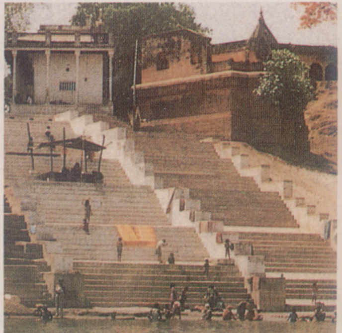
Fig 38: Renovated Oliyiar Ghat at Mirzapur
