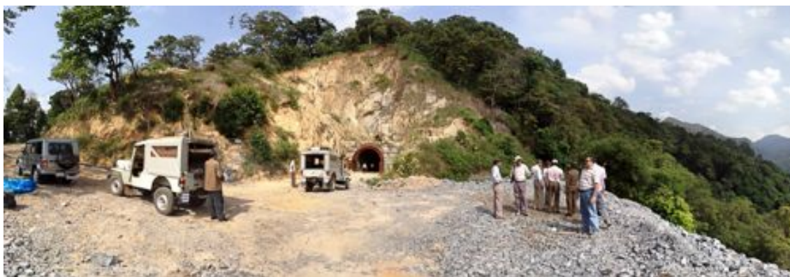
Figure 9: Tunnel blasted in a thickly forested hillock for Yadakumari mini-hydel project
