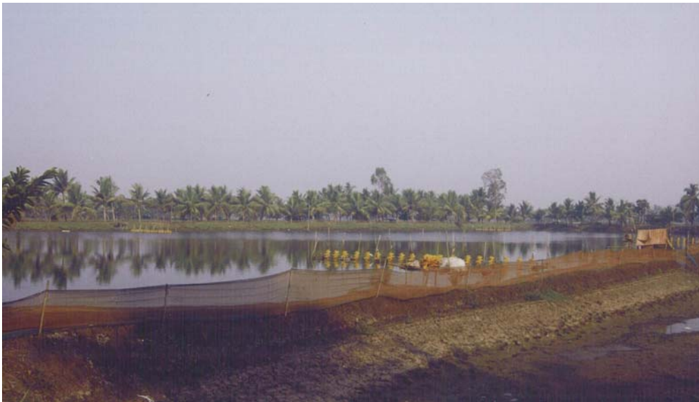
Figure 18: Embankments are made around aqua farms
