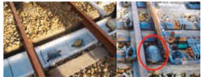
Figure 9.9. Turtle crossings installed across railway tracks by Japan Railways (left). Turtle stuck between railway tracks (right).
