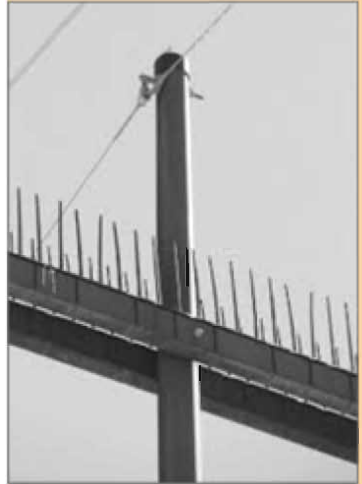
Figure 12.3. Perch deterrents are known to be effective in reducing raptor electrocutions in the USA.
