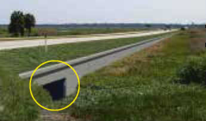
Figure 9.7. An outward lip in the wall for directing animals, especially snakes, towards underpasses.
