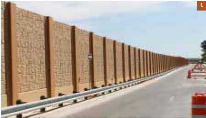
f. Cast-in-place concrete noise walls. Source: http://precast.org/2014/09/integrated-sound-wall-system/ .
