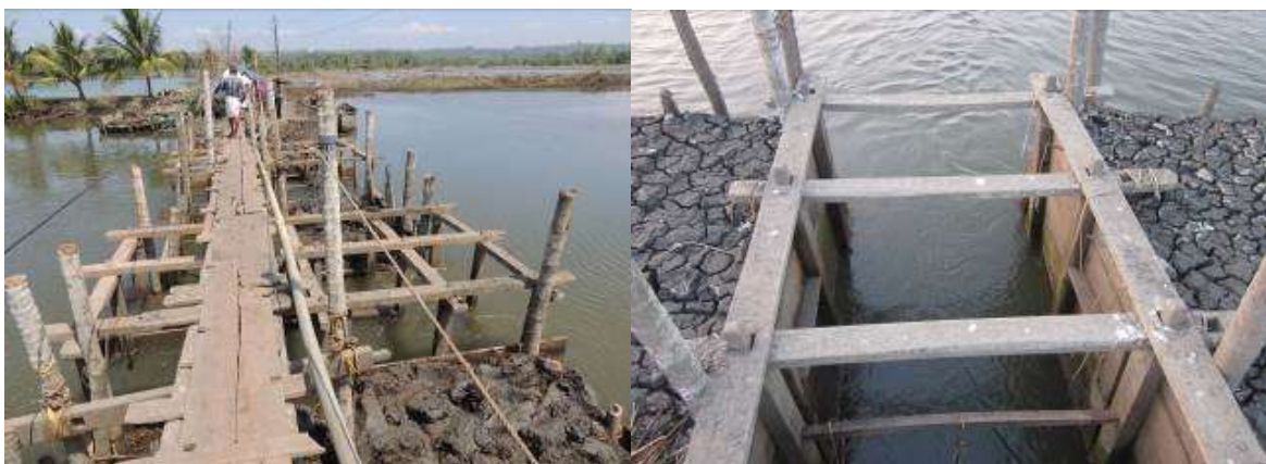
Figure 19: Sluice construction in Pokkali & Kaipad fields
